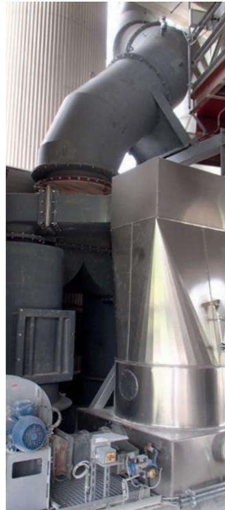
Partly visible cyclones for separation of the heated dust particles after the thermal treatment in the second preheater line
